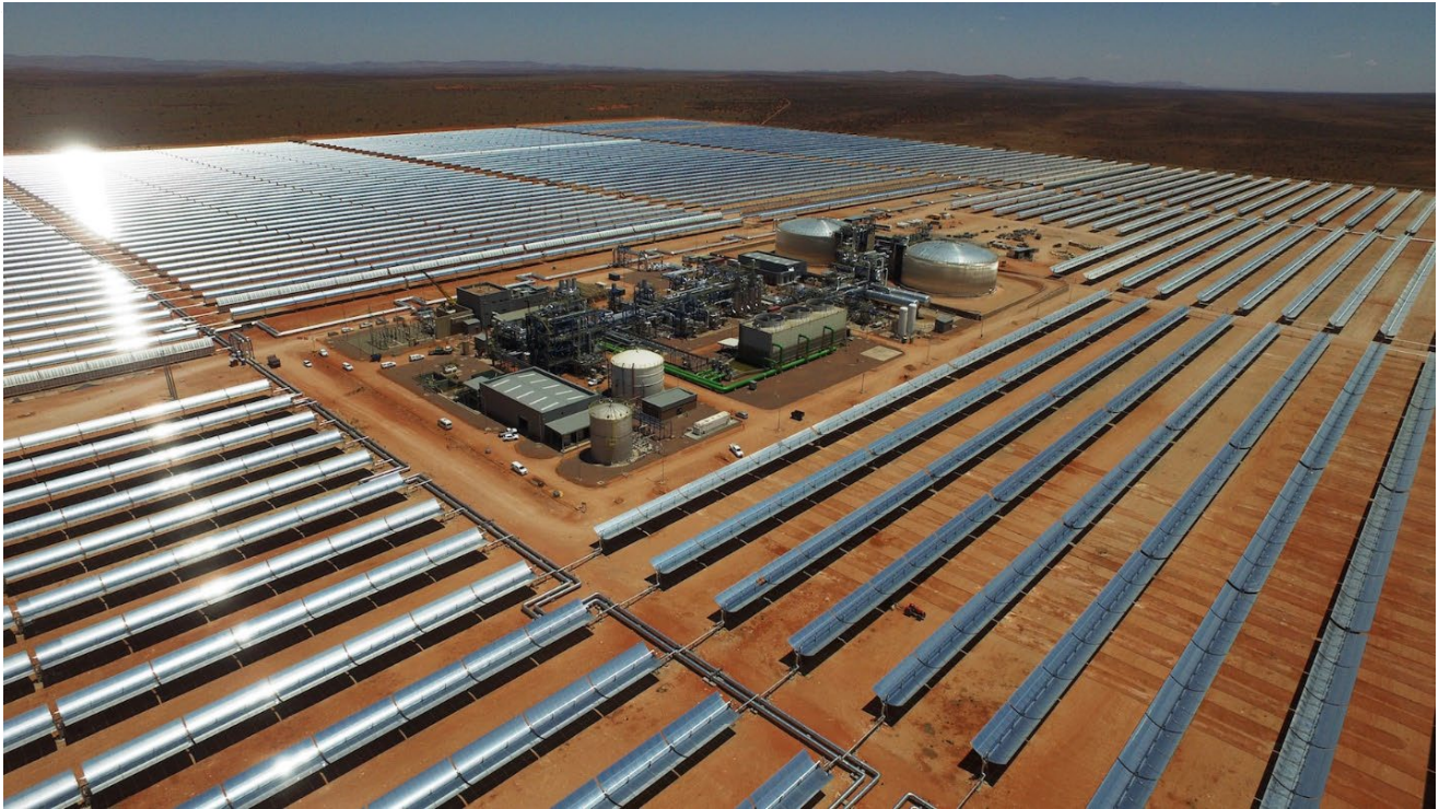
Image 2: Bokpoort Solar CSP Plant in the Northern Cape
